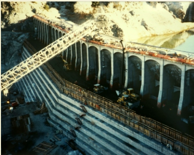
Adding Roller-Compacted Concrete
