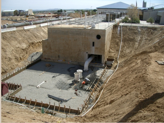
Constructing Three New Filters - 2006
