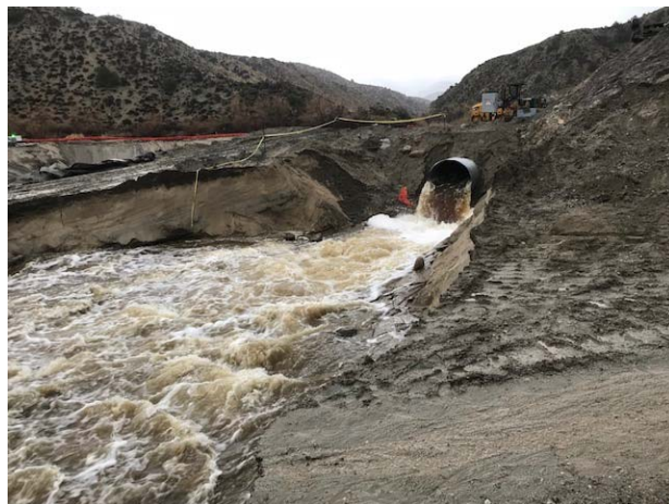
Water leaving Bypass Pipe
