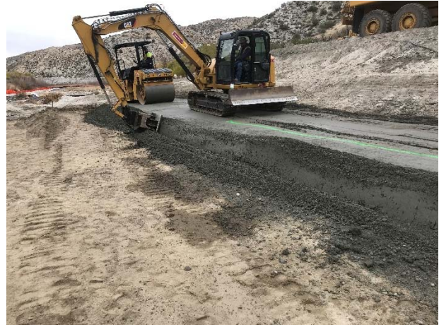
Work on RCC Test Section
