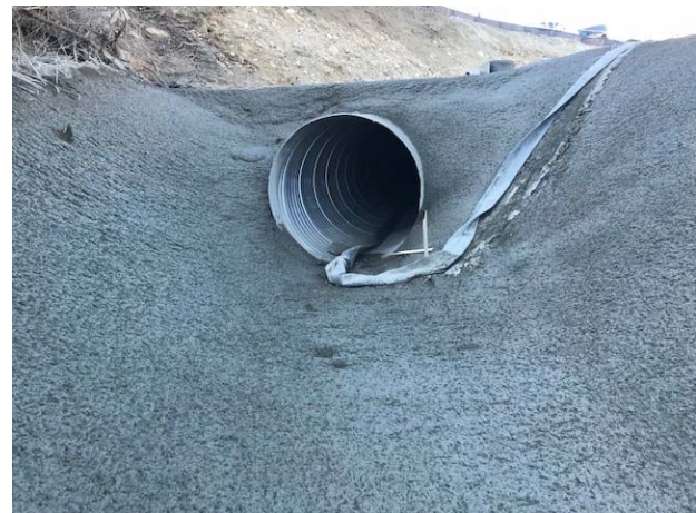
Water Bypass Pipe Installation
