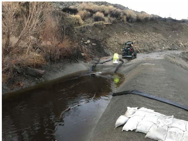
Runoff Filling Bypass Pipe Inlet
