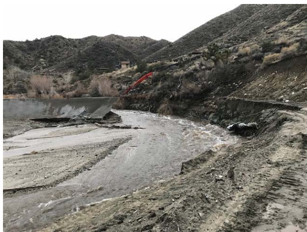
Breached Upstream Berm
