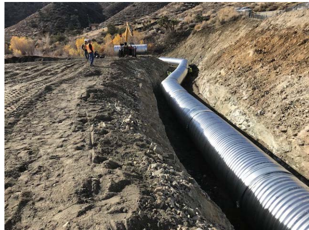
Water Bypass Pipe Installation
