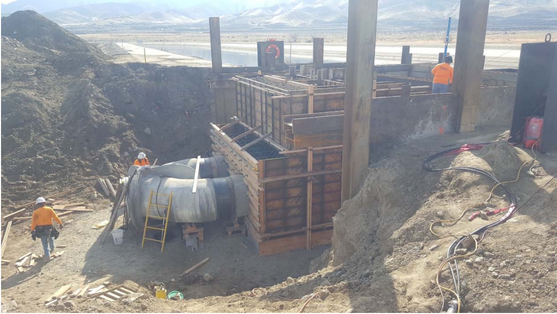
Construction of Turnout
