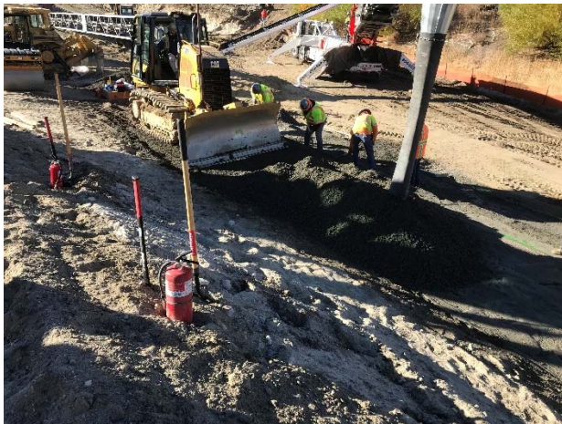
Work on RCC Test Section
