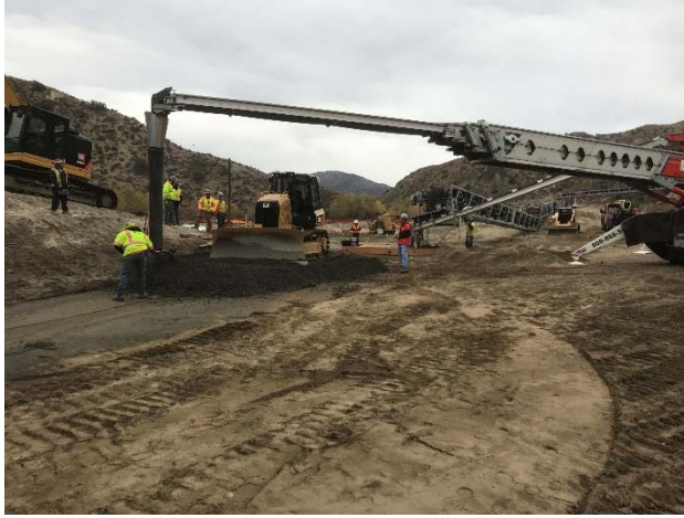
Work on RCC Test Section
