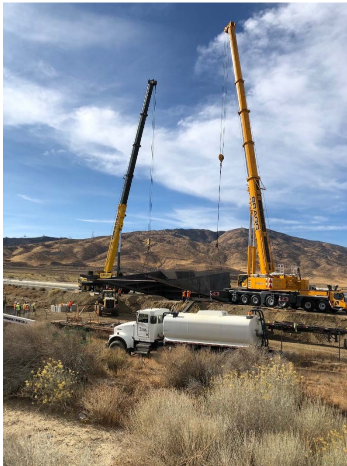
Setting Cofferdam in California Aqueduct - November 15, 2018
